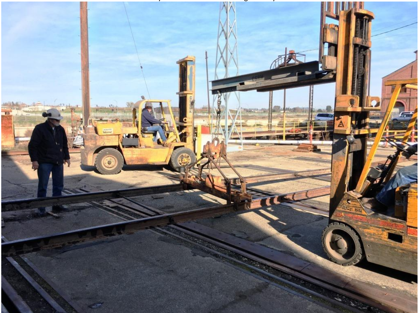
Chris uses the panel-track lifter to lift the rails and scoot them over
