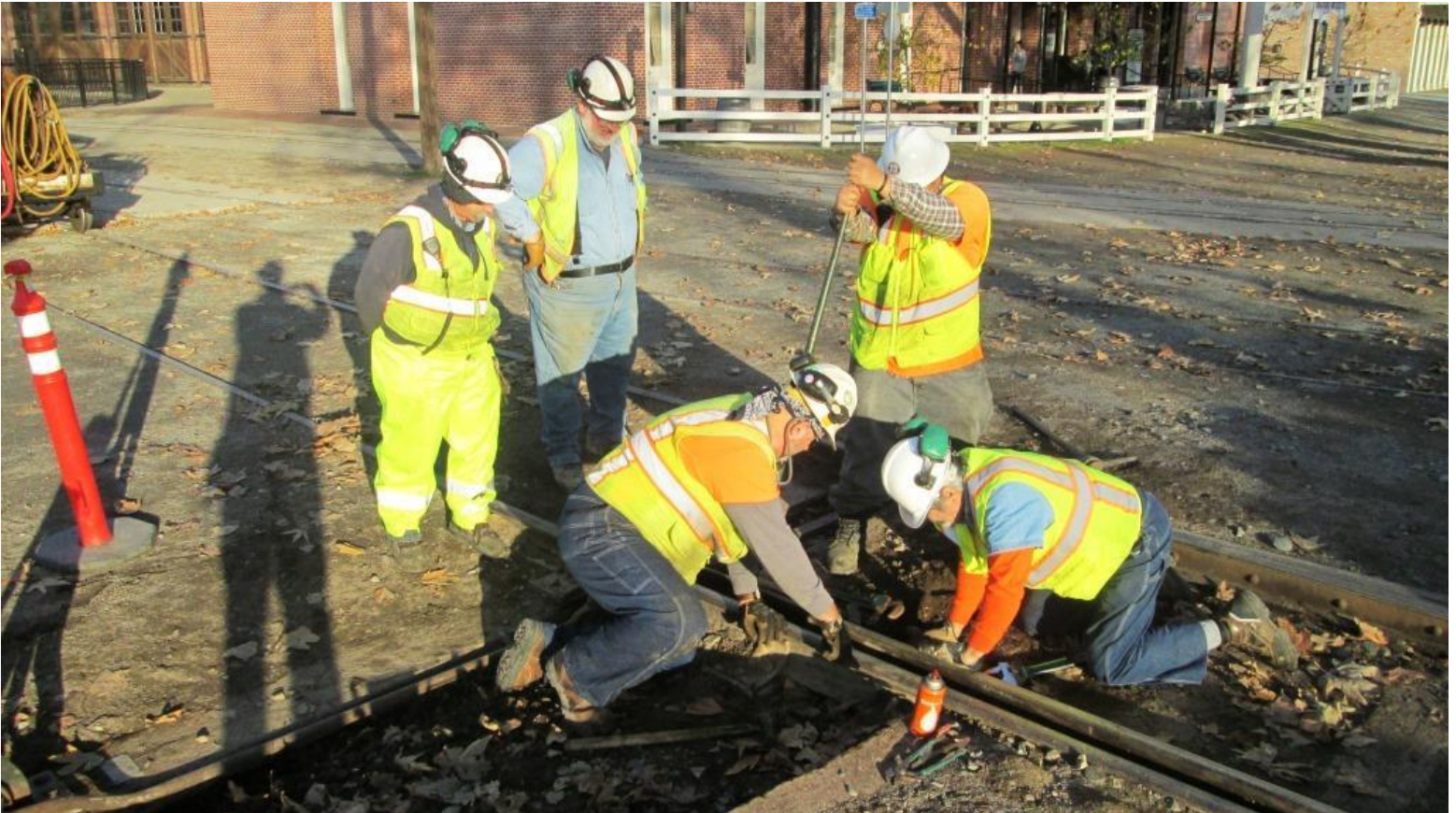
The Team makes the necessary adjustments to the switch so that it will operate correctly
