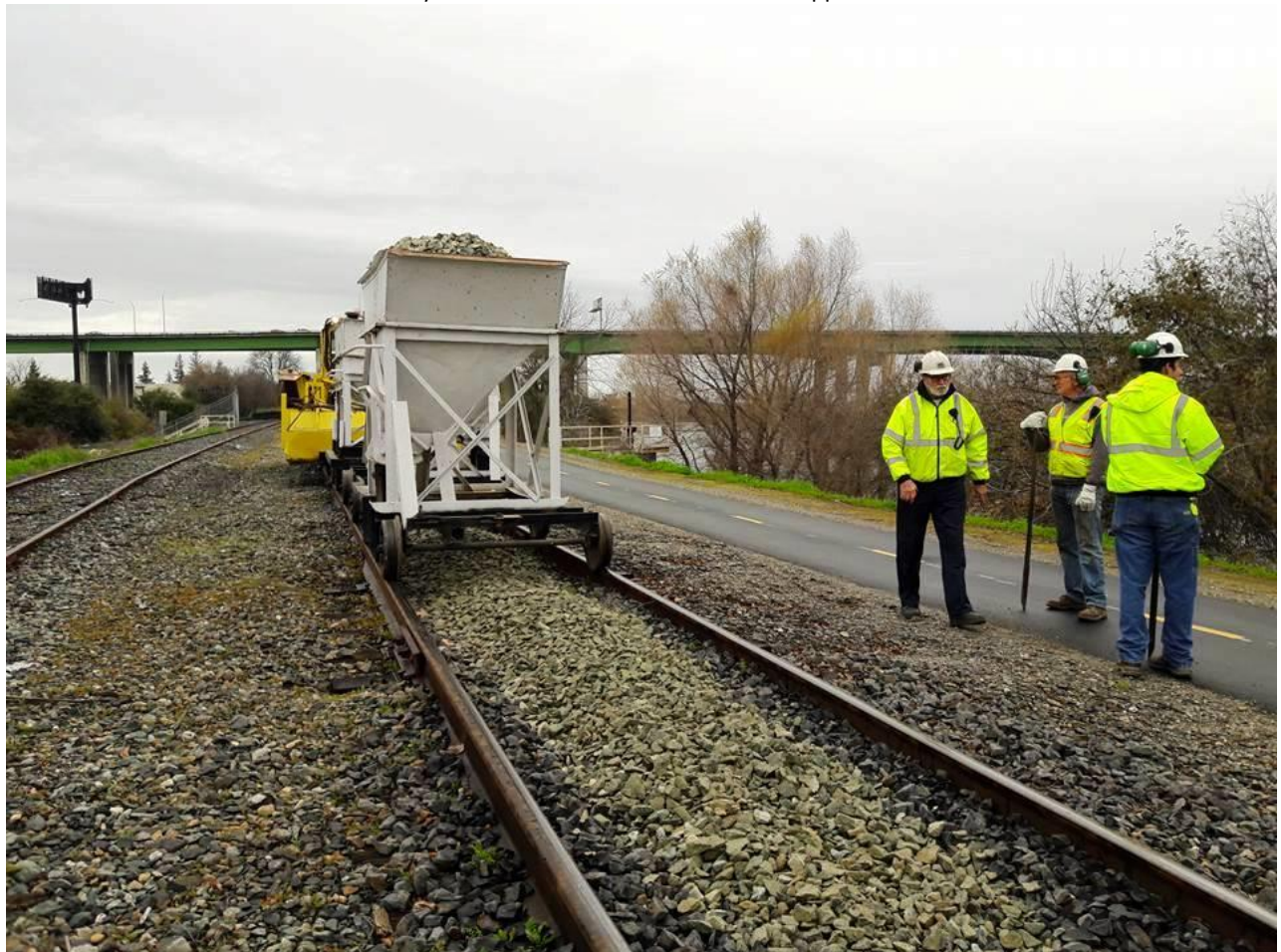
With the hoppers on site, Alan, Steve, and Weston prepare to discharge the rock
