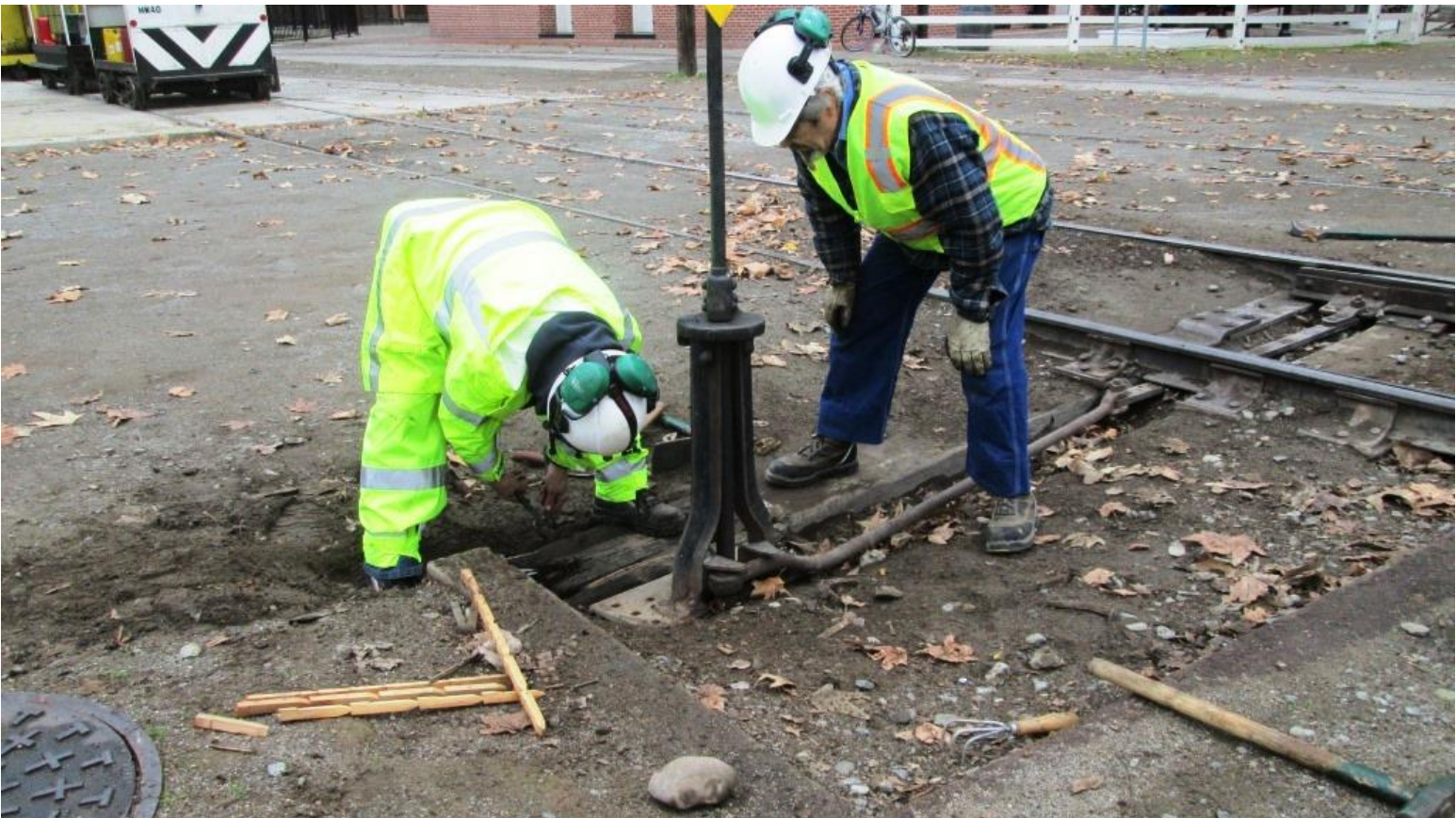
The stand is pulled to the side as Joe and Ed fill the shattered end of the head-block with wood-plugs
