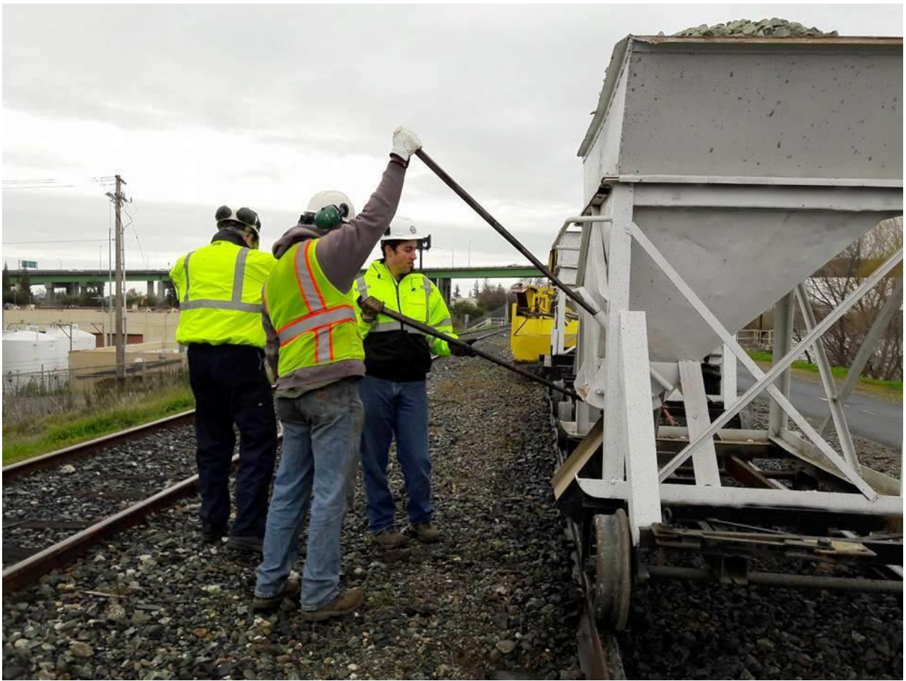
Steve and Weston drop rock along the east side of the rails
