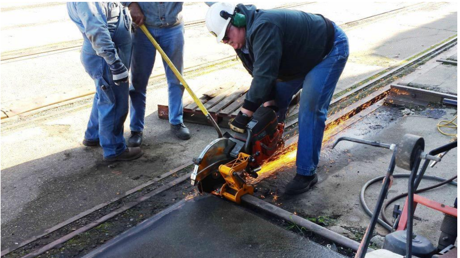
Chris uses the rail-saw to cut on the north-most Firing Line rail
