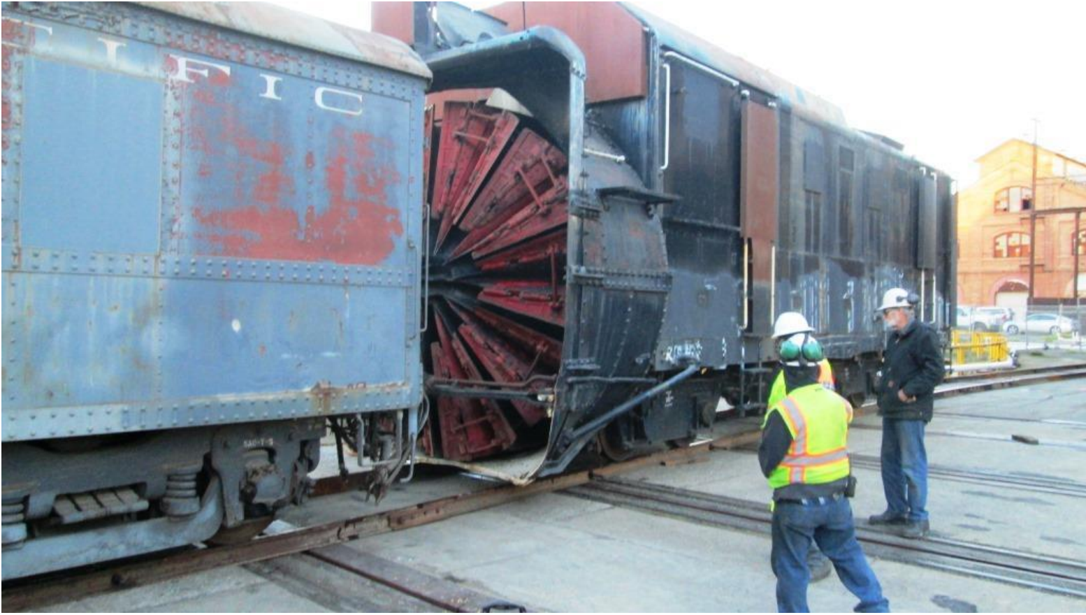
All hooked-up, the rotary moves towards the South Firing Line track
