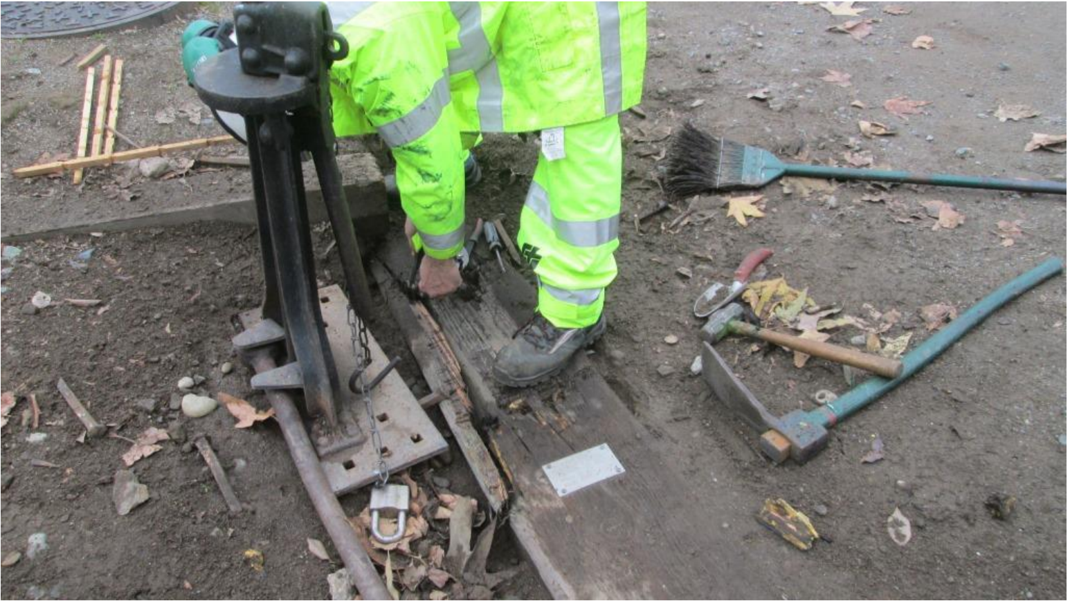
Yikes! The head-block is blown...
