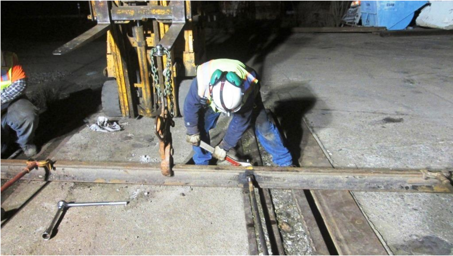
Joe tightens down a gauge-rod
