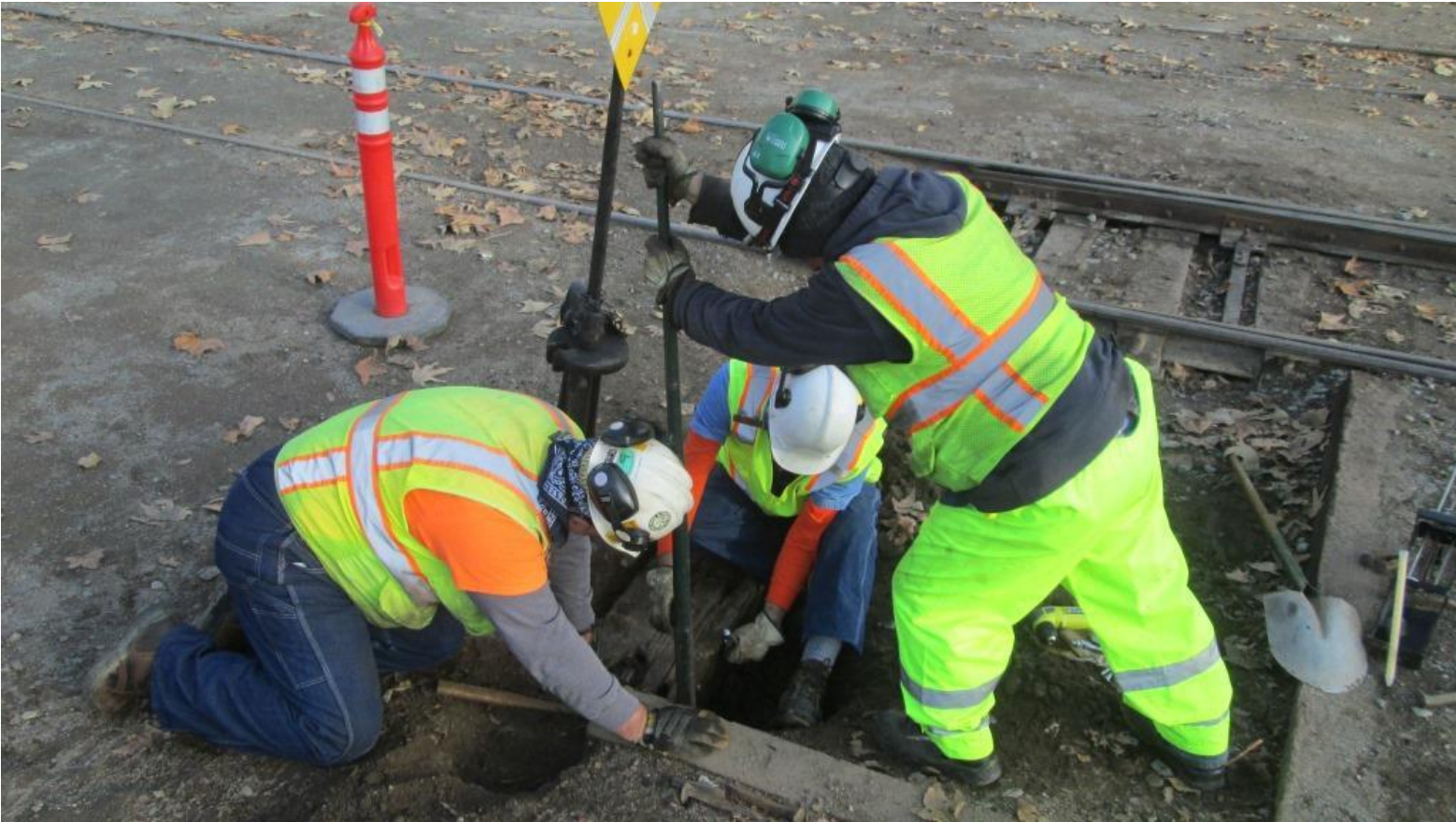
Joe uses a lining-bar to shove the split-end of the head-block closed as Mike F. and Ed bind the block with lag-screws
